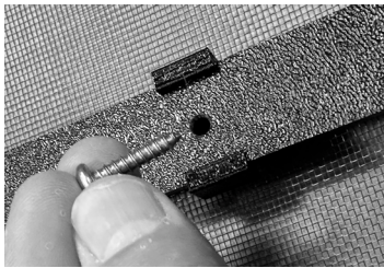
Step 10) Use Hole Screw (Z) to make a clean hole in the screen.
