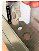
To Install Grommet: Cut "X" pattern in screen from top.
